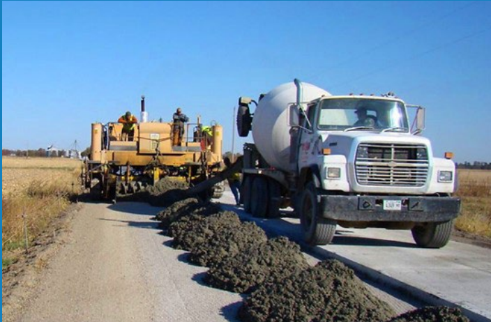
This concrete overlay was placed on County Highway 9 in Richland County, IL, in 2010. Credit: Illinois Chapter, American Concrete Pavement Association
